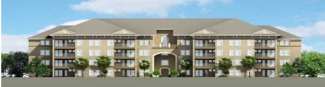
Gateway Village 4-Story Building
